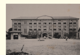
1921(大正10)年、麹町区元衛町1番地に完成した新校舎 In 1921, new school building completed at 1 Motoe-cho, Kojimachi-ku, Tokyo.
