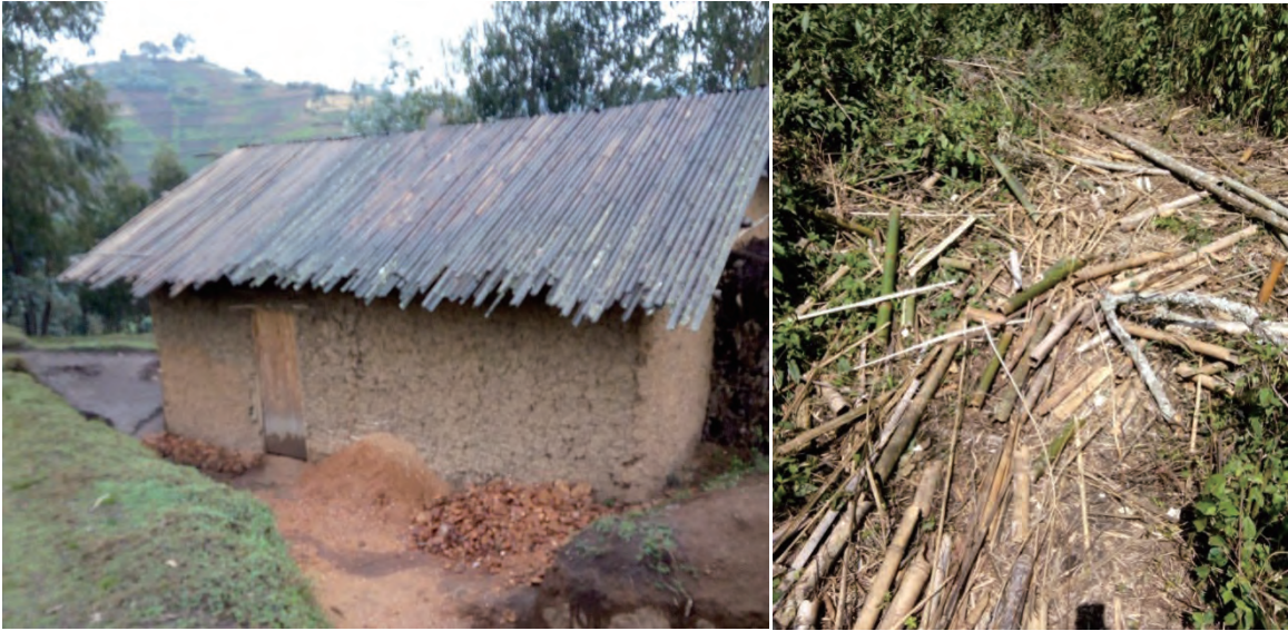
Figure 3. (left) Bamboo used to build roofs on some houses; (right) bamboo parts are left inside the bamboo forest zone.
